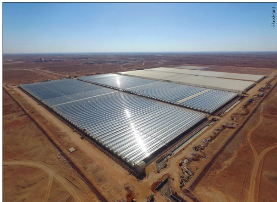
Aerial view of the huge greenhouses protecting the steam-generating mirrors at PDO's Miraah EOR project in Oman: an example of an NOC using renewable energy sources to reduce its emissions due to E&P operations.
